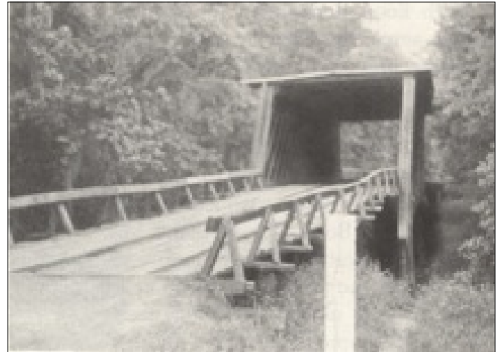
Covered bridge over Pintlala Creek on Wasden Road, undated photo, from Montgomery Advertiser
